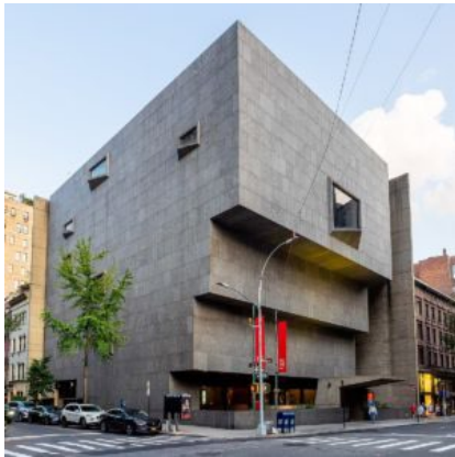
945 Madison Avenue, also known as the Breuer Building
