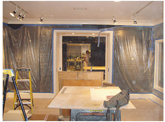
Center Gallery Looking Towards Storage Room
