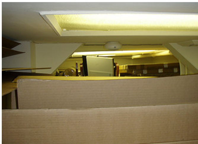
Storage Room – Looking Over the Top
