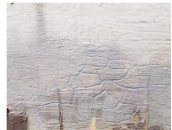
Another very similar problem is referred to as **alligatoring**. As the names suggest, the appearance of these cracks is much like the skin of an alligator ... wide areas where the paint surface, during the drying process, has shrunk and the lower layer is visible.
